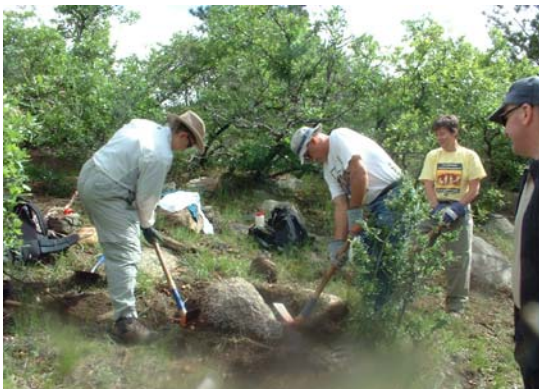
Volunteers moving boulders during the VOC Trail Building Event in June 2005
