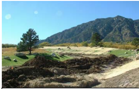
Utilities being laid in the campground.
